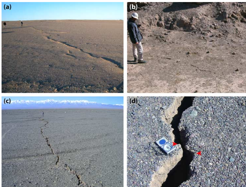
Figure 2. Field observations of surface faulting features. Locations and orientations of the photographs are given in Figure 1. (a) Surface rupture north of Bam with en-echelon pattern; (b) Cracking at the foot of the ridge visible in the ASTER image west of Baravat; (c) View southward over en-echelon patterns of surface rupture on the main seismogenic fault south of Bam; (d) Close-up at the locality shown in (c), with right lateral displacement of \sim 20 cm.
